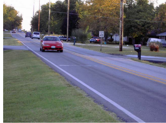
Illustration 3. Lack of pedestrian and bicycles facilities on a 45 mph road, in a residential area of Battlefield, MO.
