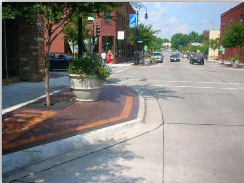
Downtown Lee’s Summit: Bulb outs and cross-walks make the downtown more livable.
