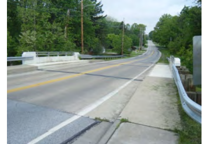
Looking west at Martin Ave bridge
